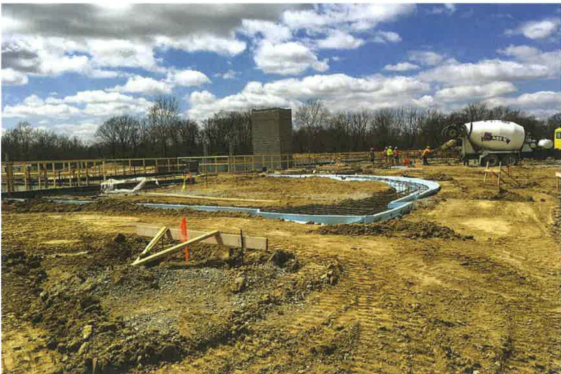
Upper Level Footings
