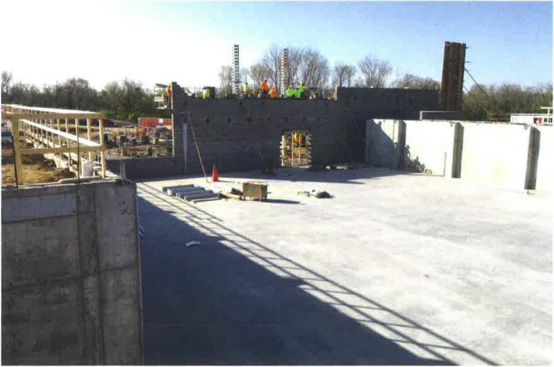
West Natatorium Wall
