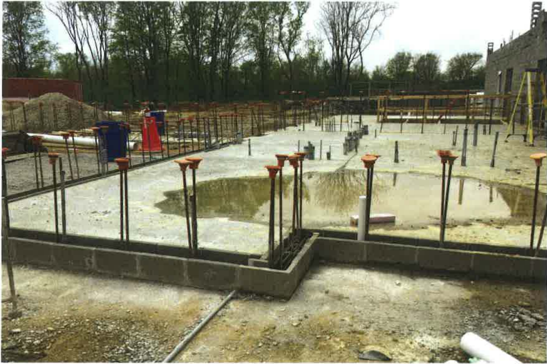
Electrical and Pool Mechanical Room Slabs
