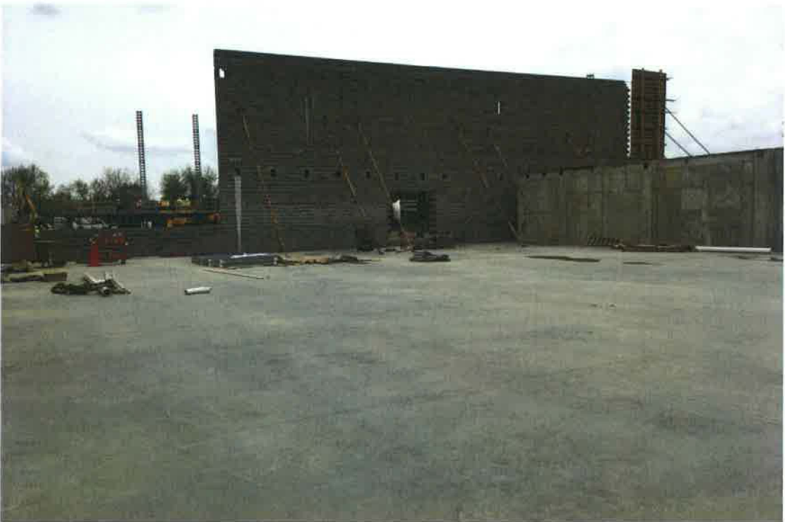
West Natatorium Wall
