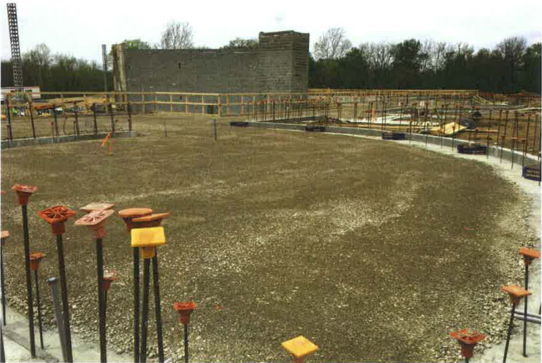
Upper Level Building Pad
